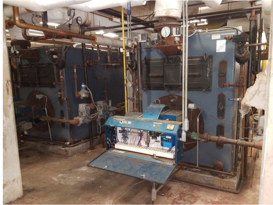
Dows Lane Boiler - Failing pipes and sessions
