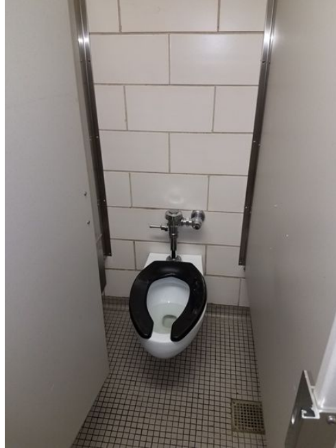
HS Girls Bathroom - Renovation Needed
