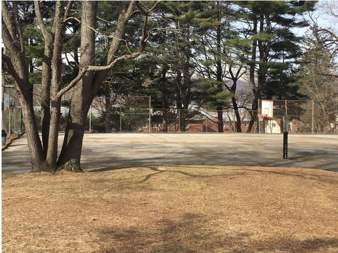
Repave Basketball court
