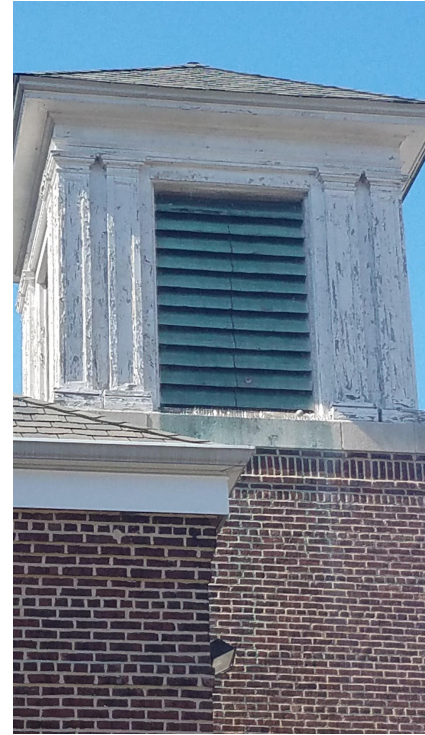
Repaint Main Street School Bell Tower
